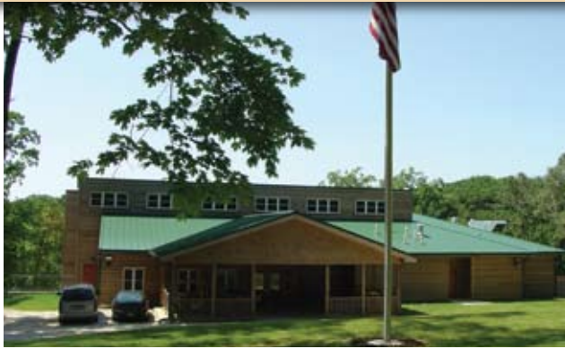
Complete with a large lobby, commercial kitchen, nine guest rooms, laundry facilities, an office, and meeting rooms, Lakeview Lodge is the center for Camp Akita activities.
