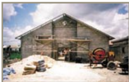
Maranatha teen volunteers helped build this church at Villa Cerro, Dominican Republic.
