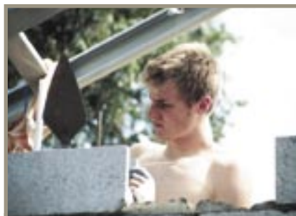
Jermey Weaver lays block on the new church building.
