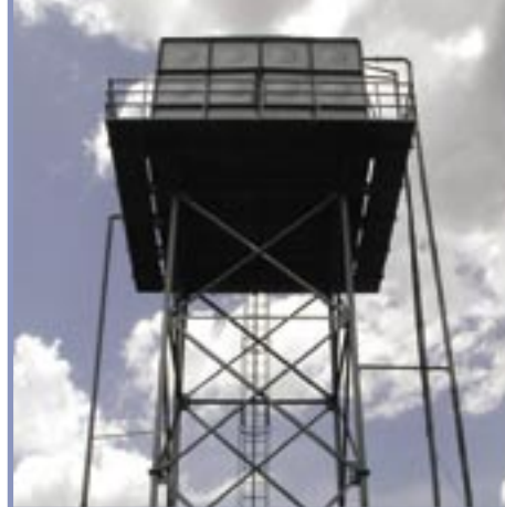
The school water-treatment plant is outdated and inadequate for the school and community’s needs. This is the water tower for the current aging water system.
