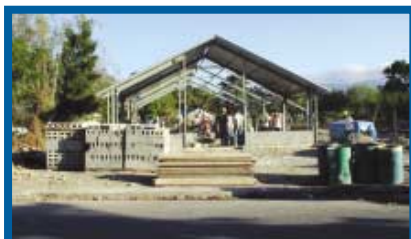
The church building begins to take shape, bringing joy and satisfaction to the hard-working SOW (Service, Outreach, Witness) Safari workers.
