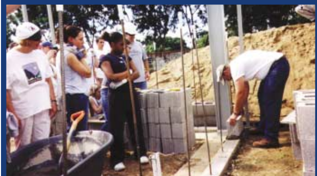
Richard Spencer, project building supervisor, lays the first block of the new church.
