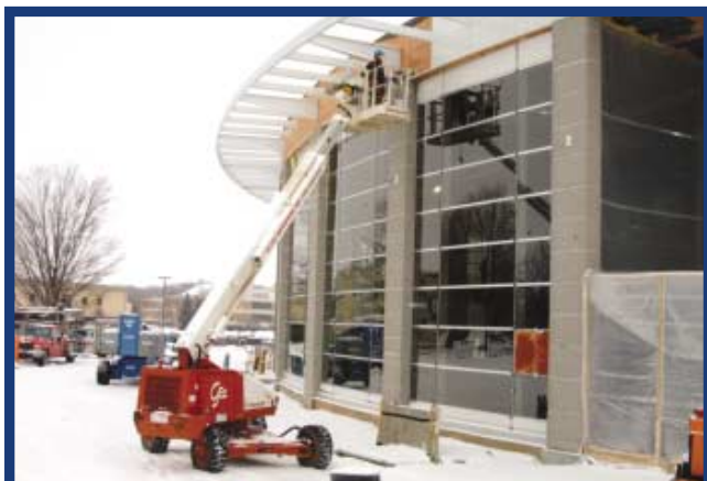
Construction on the Howard Performing Arts Center continues in spite of cold weather and snow.
