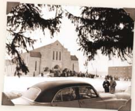
Photographed in 1959, the newly constructed Pioneer Memorial Church during its first winter season
