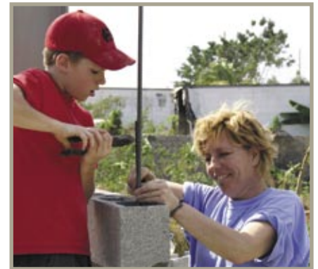
Cody Miller and Colleen Asmussen tie rebar together.
