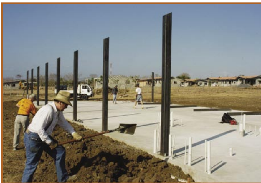
Ben McCash of the Hinsdale Church works on the construction of the new Adventist church in Las Tablas, Panama.
