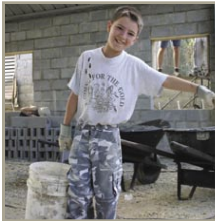
Patrick Hug carries everything at the job site, including heavy buckets of mortar.
