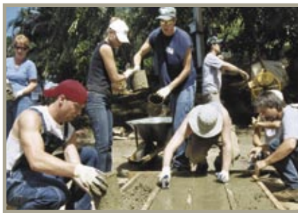
BCA students Jacob Bishop, Deni Conkell, Troy Kossick, and Roni Fogg pour and finish concrete for the amphitheater benches.
