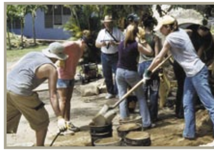
Laura Eastman shovels sand for the concrete.
