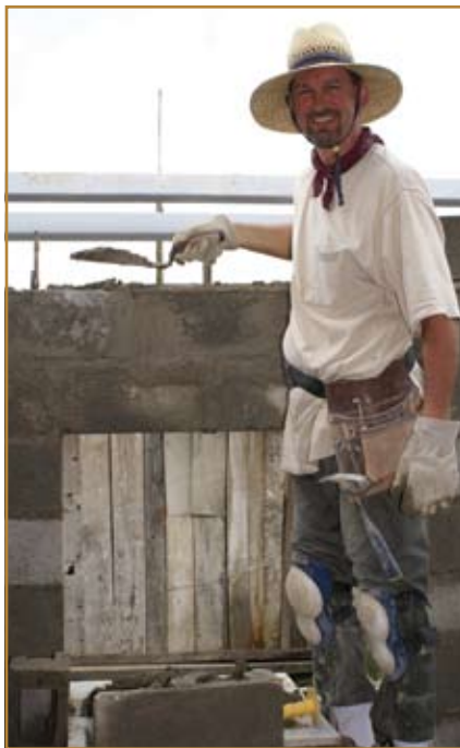
Jim Today helped build two churches while on the mission trip. The group held a special service in the church at the end of the week to celebrate the construction project being completed.
