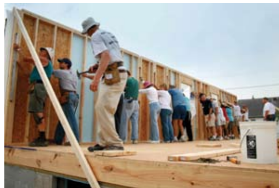
Eastminster Presbyterian Church members joined forces to raise the first wall of the Apostle Build house the first Saturday of the project. Evansville Adventists will also play an important role in the house's construction by installing drywall mid-week instead of on Sabbath.
