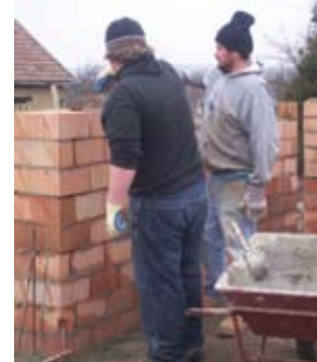
Nathan Lowry and senior parent Steve Martin laid brick for the walls of the new church.
