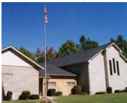
Muncie Church with new sanctuary addition on the right
