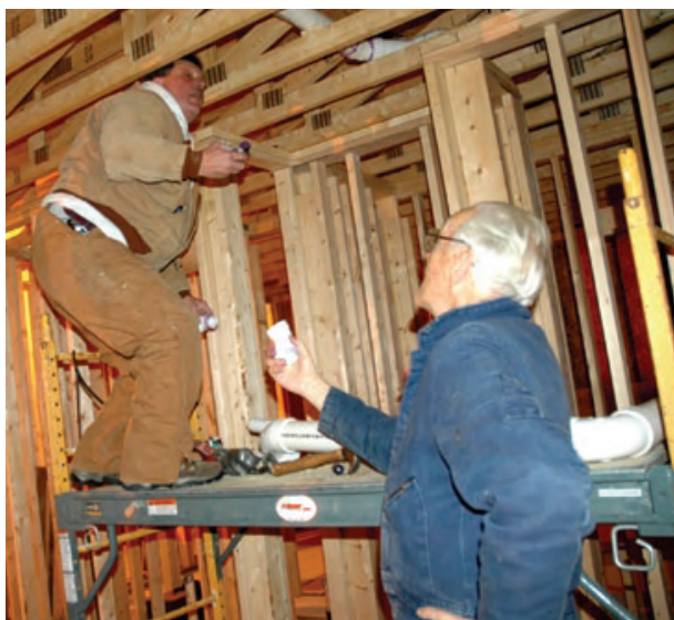
Volunteers Carl Norris and Arthur Weaver install plumbing in Deer Lodge.
