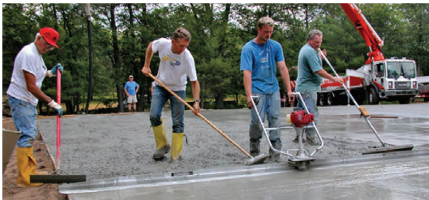
Volunteers have worked hard to complete the new Pathfinder Pavilion for the August camporee.
