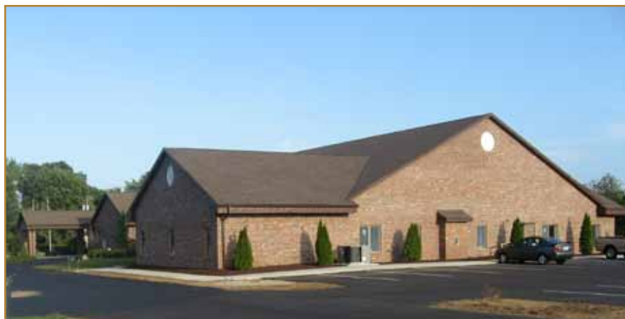
The new Education Wing added to the back of the Michiana Fil-Am Church houses a church office, two Sabbath school classrooms, a youth room and a conference room.
