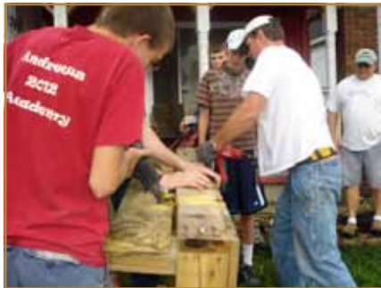
Nineteen young people from the Junior, Earliteen and Youth classes, along with ten adults, came together to help build a wheelchair ramp for a family in their community. They also painted a mural in the boy's room, and did some yard work at a neighbor's house.
