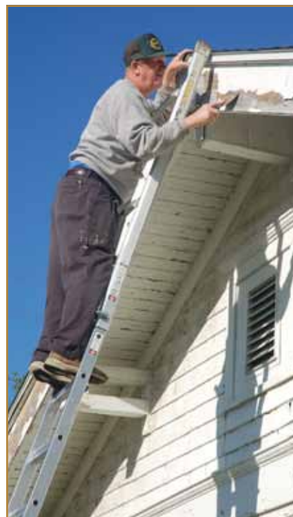
SAGE volunteer Bob Jones tackles the tedious task of scraping and removing old peeling paint to ready this building for a face lift.
