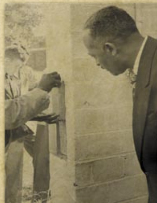
Rothacker Smith inspects work on the church building in Benton Harbor.
