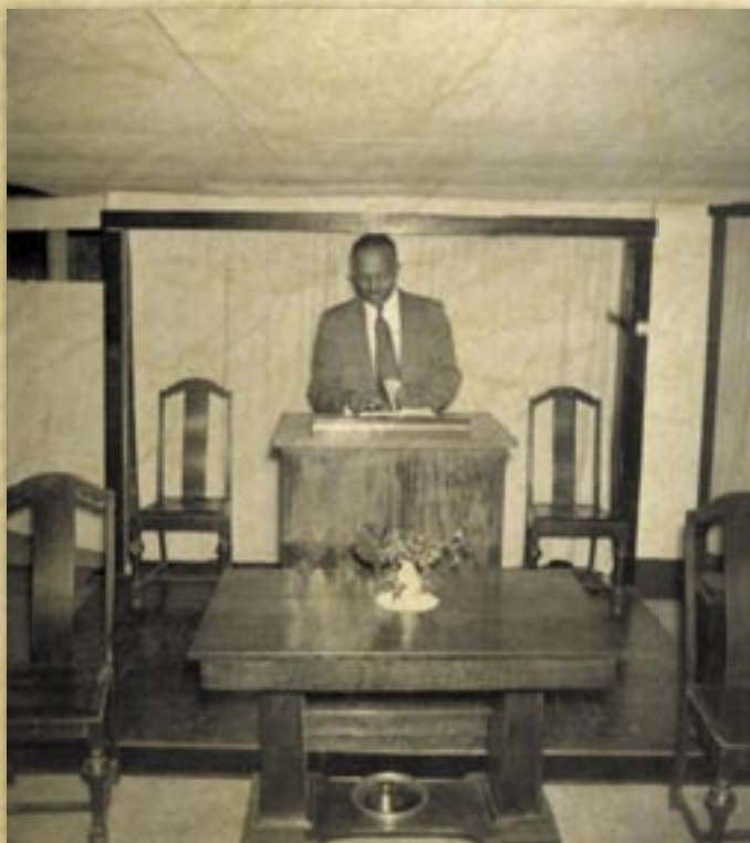
The basement of the under-construction Main Street church served as the sanctuary for almost two years.
