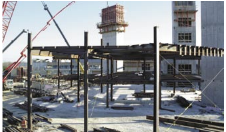
Steel girders are going up on the Adventist La Grange Memorial Hospital Patient Care Center, which is anticipated to open in June 2006.
