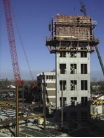
Adventist La Grange Memorial Hospital is building a new Patient Care Center, but that's not all that's under construction there.
